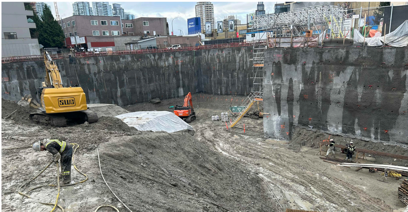
April 09, 2025: View of the west side. Scaffold stairs installed to facilitate crew access to the excavation area.
