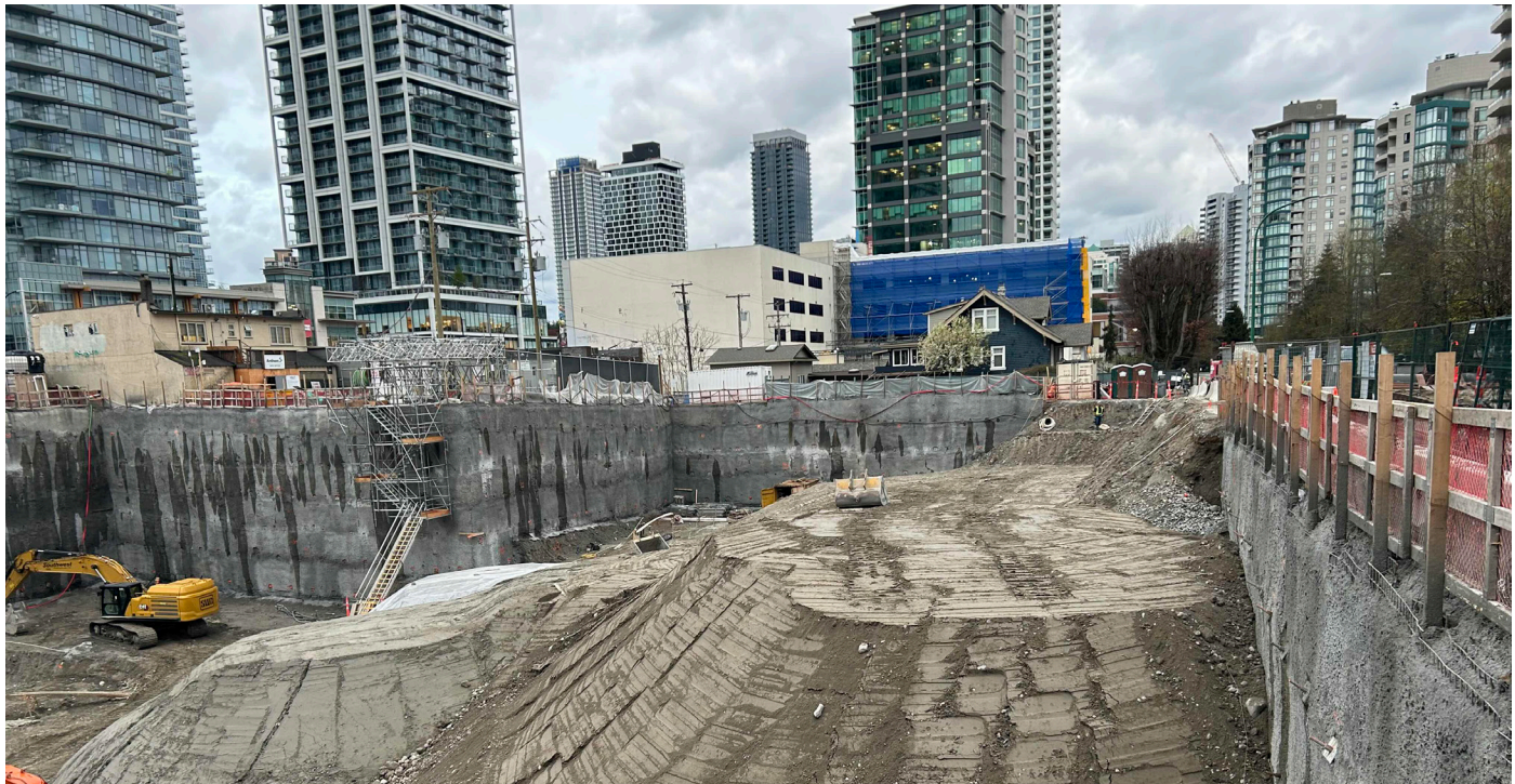
April 10, 2025: Looking north across the Citizen site – crews working along the north shoring wall and access route. Shoring the 1st row on North side.
