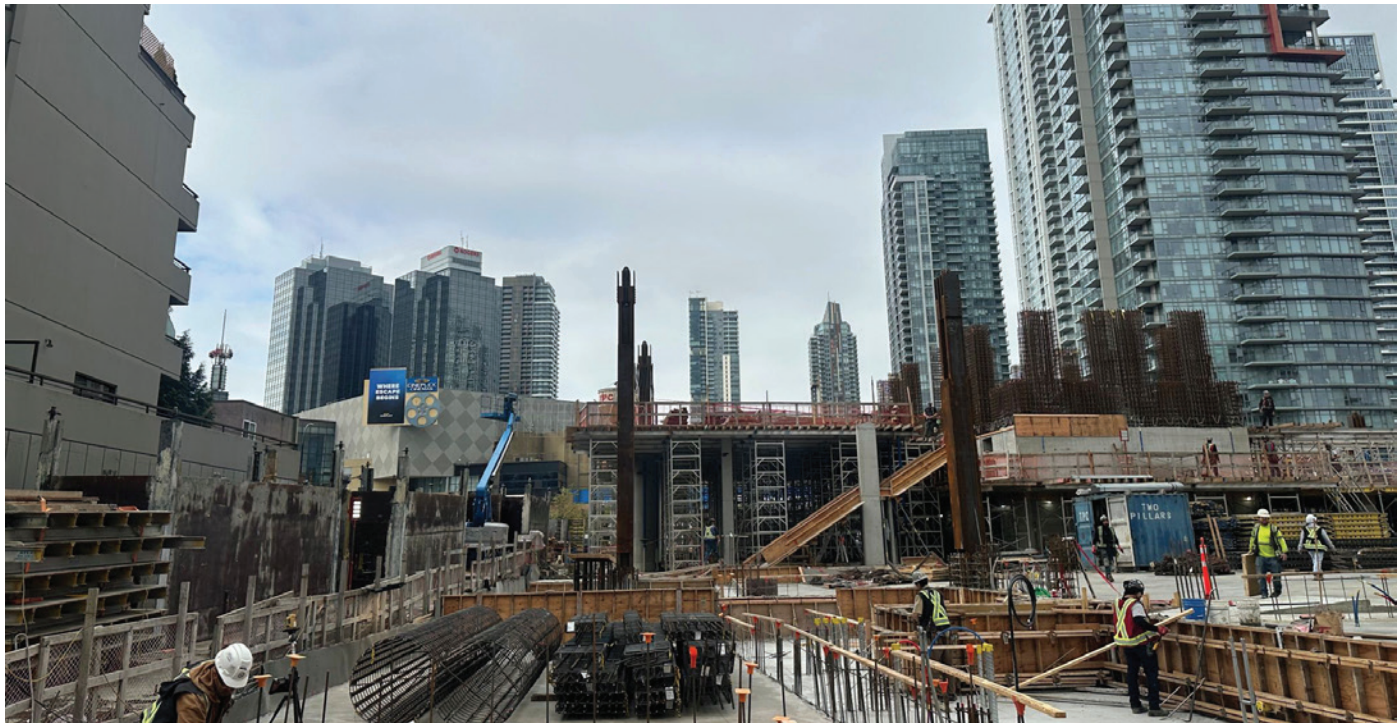
May 11, 2026: Shot from L1 slab looking towards the Southeast L3 formwork.
