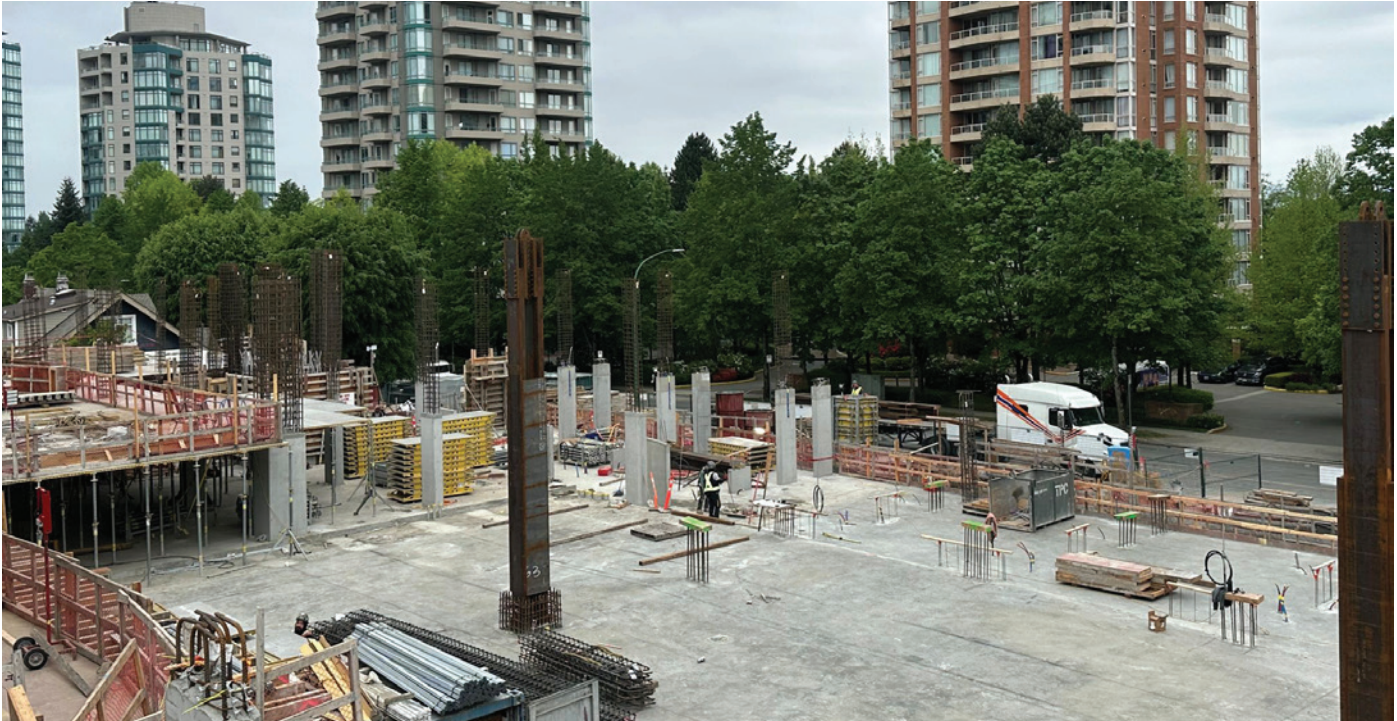
May 11 2026: level 1 Slab looking across the future covered loading area from the dedicated future road on the Eastside of the site.
