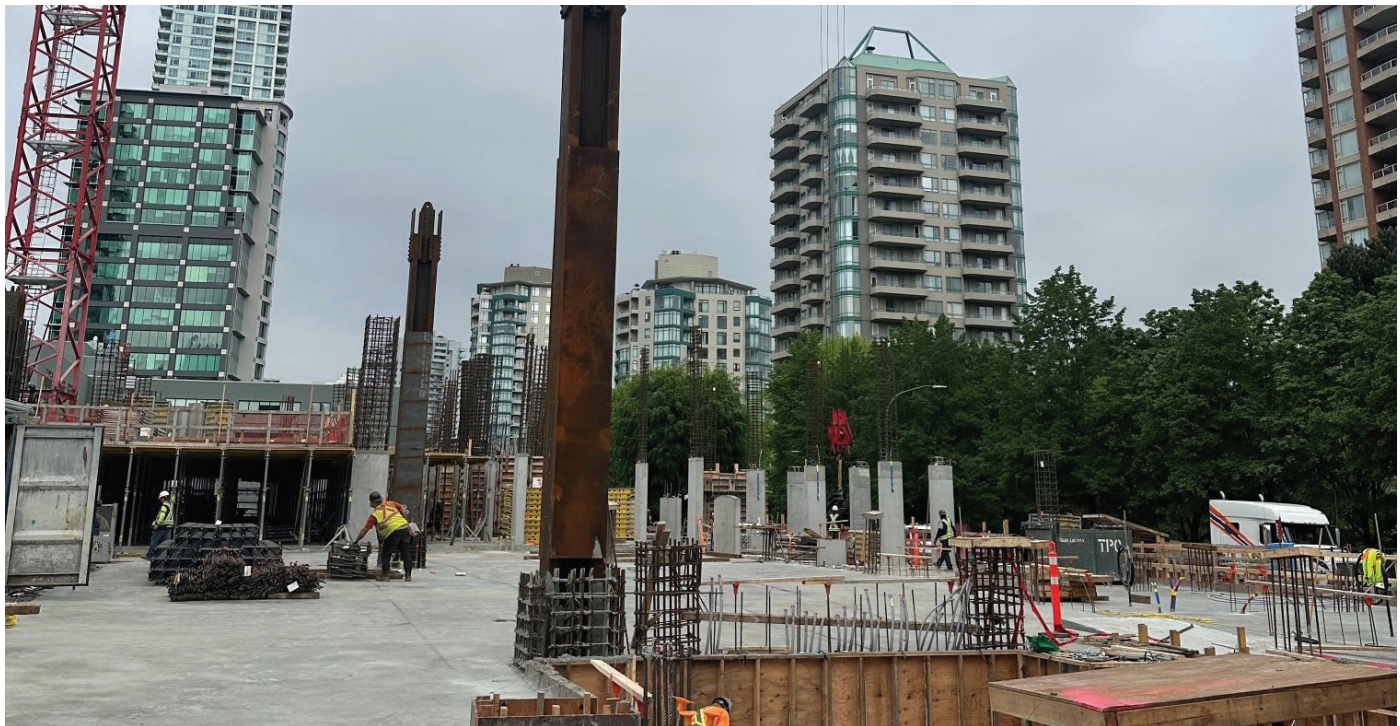
May 11, 2026: Level 1 Slab looking west towards parkade entrance on Hazel Street.
