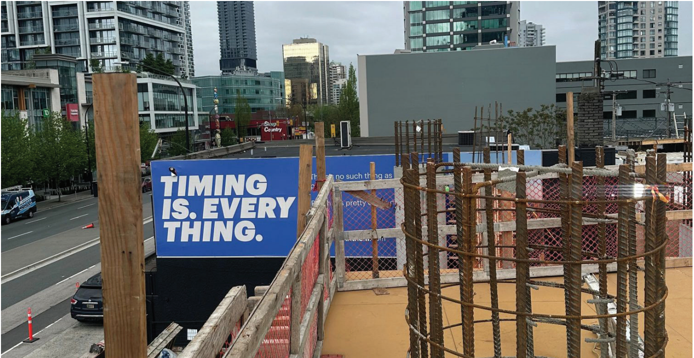
May 11 2026: Column on level 3 near Kingsway.
